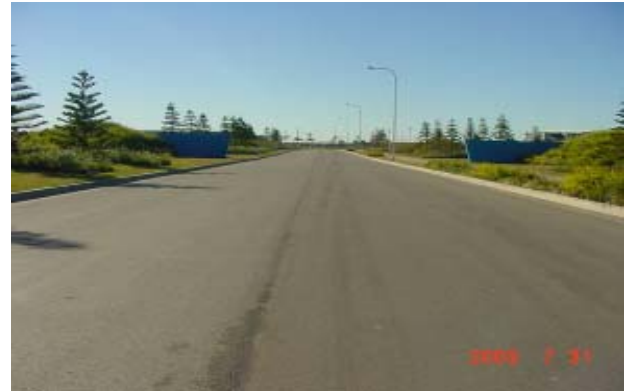
After rigorous analysis, Cardno MBK chose XP-SWMM for the Kawana Waters project due to the model's ability to simultaneously and dynamically model both the surface and piped drainage systems.
